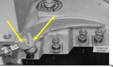
IF USED, PLACE JUMPER- P/N 10532508 -ON TOP OF BATTERY CABLE
